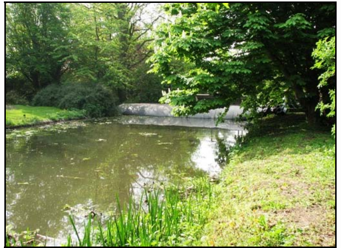
Picture 3: Upstream of the AquaDam in the River Colne, showing the level of water retained (around 1.2 metres deep). (NE Thames Operations Delivery)
